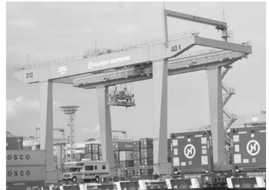
写真7：Automated Rail Mounted Gantry Crane
